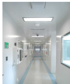
Rova 126 Slab Ceiling installation.
