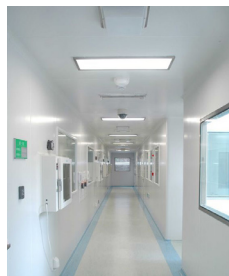
Rova 126 Slab Ceiling installation.
